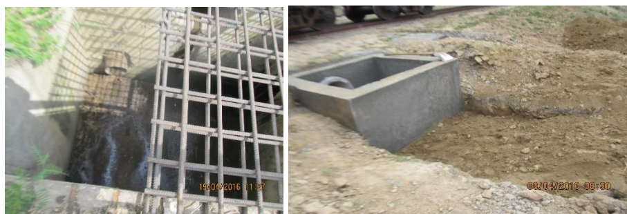
Photo 2: Passage corridor for reptiles and amphibians, and other small species
