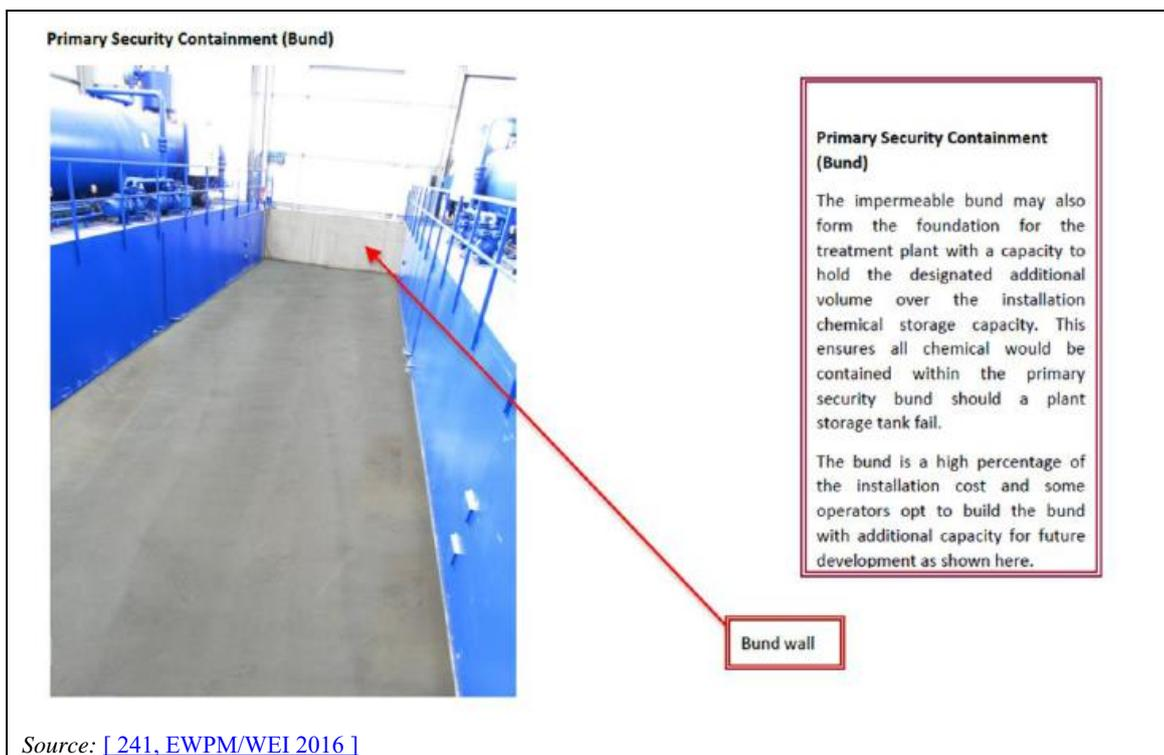
Figure 15.21: Design examples for process containment
