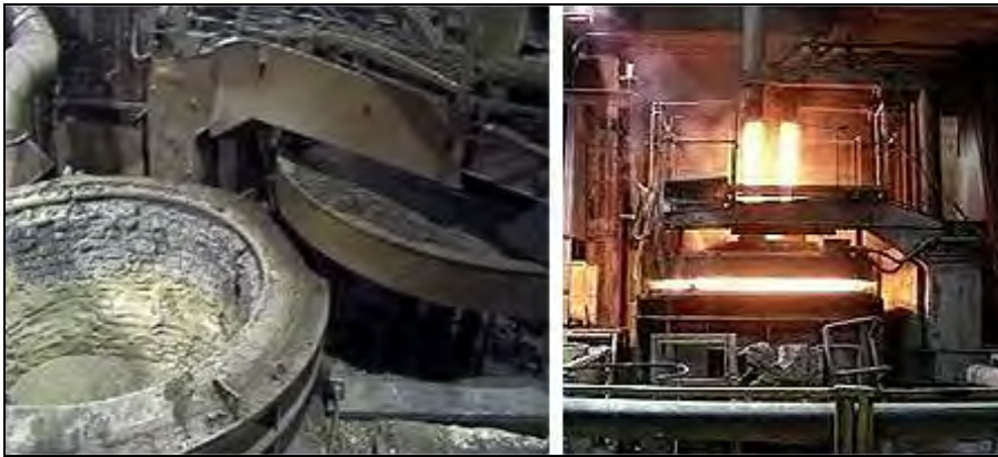
Figure 2.12: EAF furnace [237, HUT, 2003]
