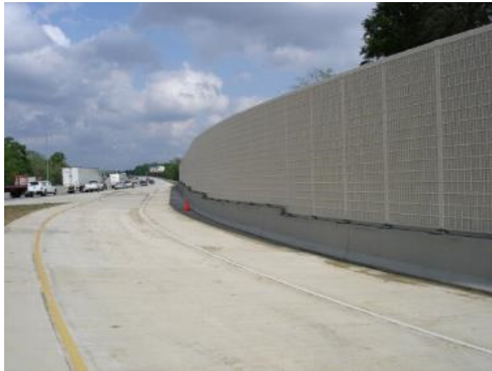
Figure no.7-6 Example of sound-absorbing panels recommended for the Suceava DN2H highway and the Siret border DN2H expressway
