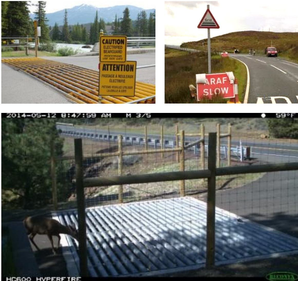
Figure no.7-3A. Example of an electrified wildlife fence; B Example of a warning sign on a road in Wales to alert drivers to the presence of a grating; C. Fence installed to keep wildlife out of the roadway on a road in Washington, USA
