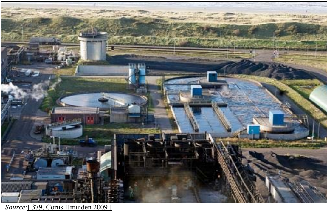
Figure 5.24: Aerial view of the biological waste water treatment plant at Corus, IJmuiden, the Netherlands
